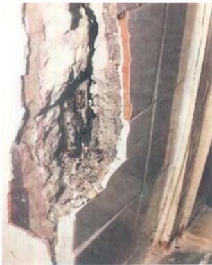
Main Bathroom Reinforcement corrosion and spalling of column.
