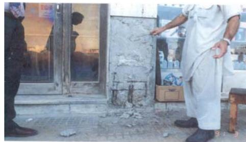
Corroded Re-inforcement in Column at the front
