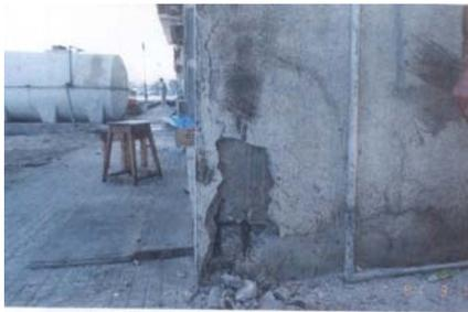
Corroded reinforcement in the Ground Floor Column at the corner
