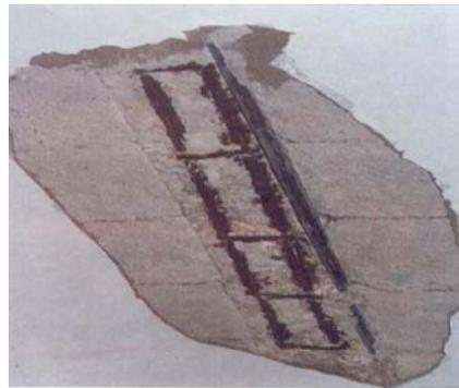
Severely corroded reinforcement
